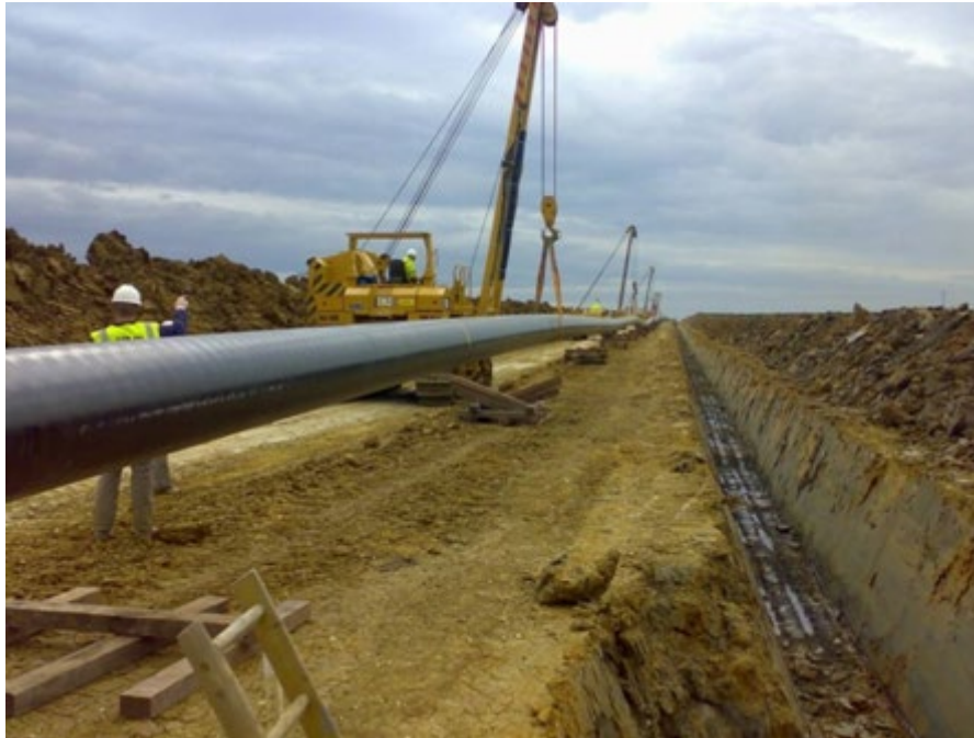
Figure 6-4 - Lowering pipe into a prepared trench
